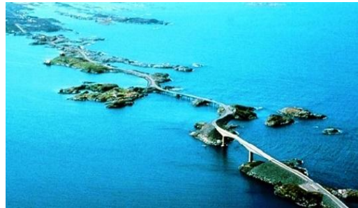
Slika projekta Coastal Highway Route 1
